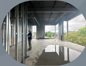
3 rd Floor Fireside Room
