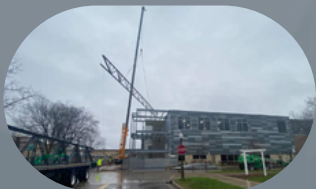
Roof grider supports installed
