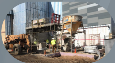
Elevator Shaft Install
