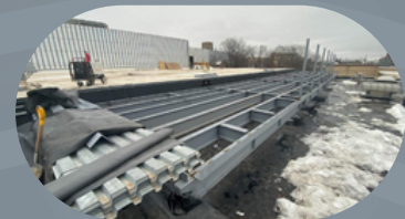
3 rd floor patio supports
