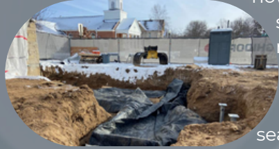
Foundations & footings prepped for concrete
