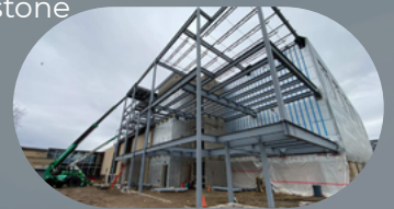
Exterior supports installed
