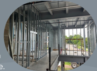
2 nd Floor Office Spaces
